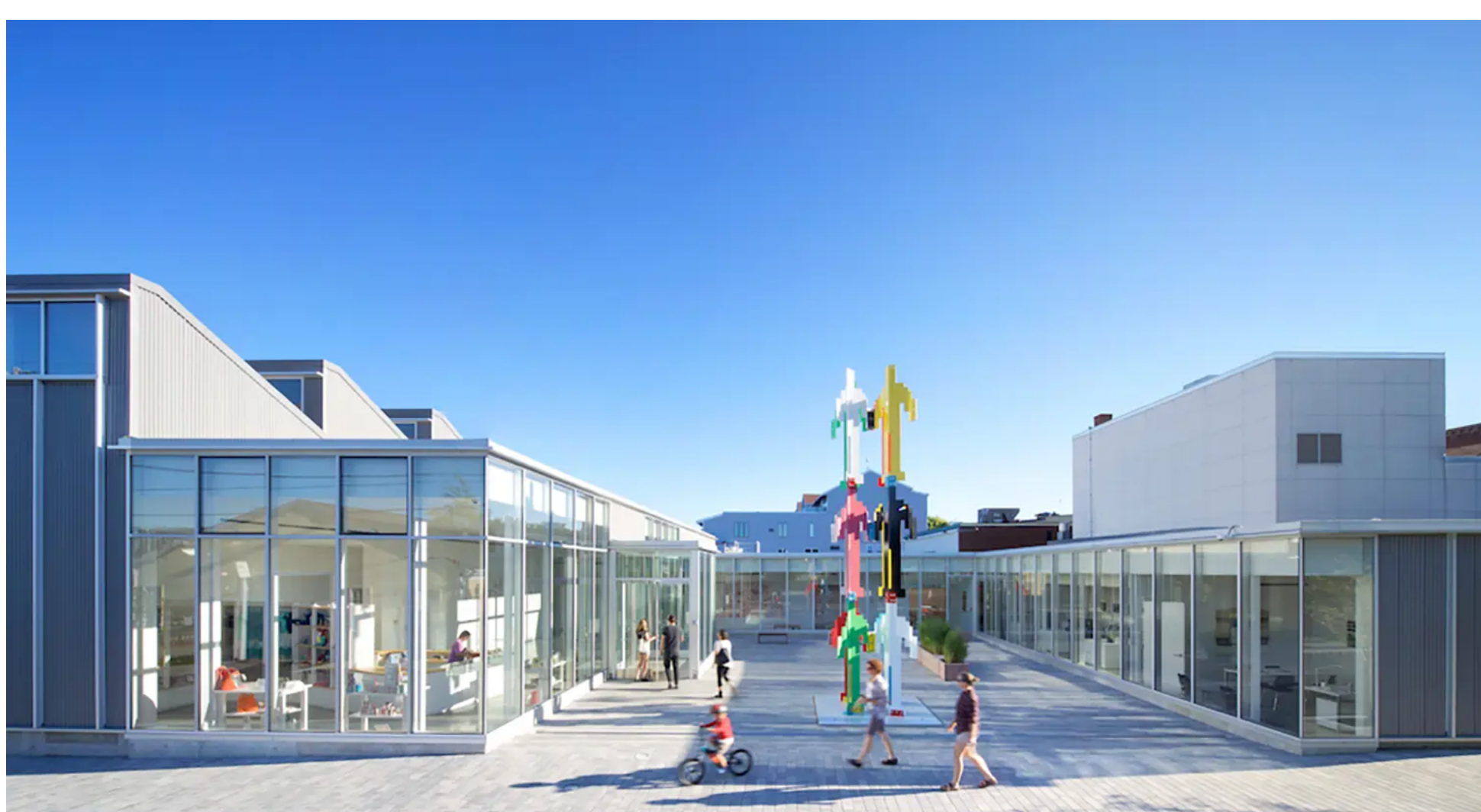
The Center for Maine Contemporary Art and its courtyard, designed by Toshiko Mori in 2016
